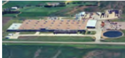
Hoisington Communications Plant | Hoisington, KS
