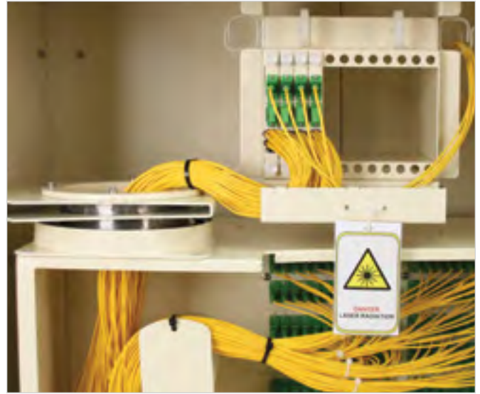
Fiber Management and Bend Radius Control
